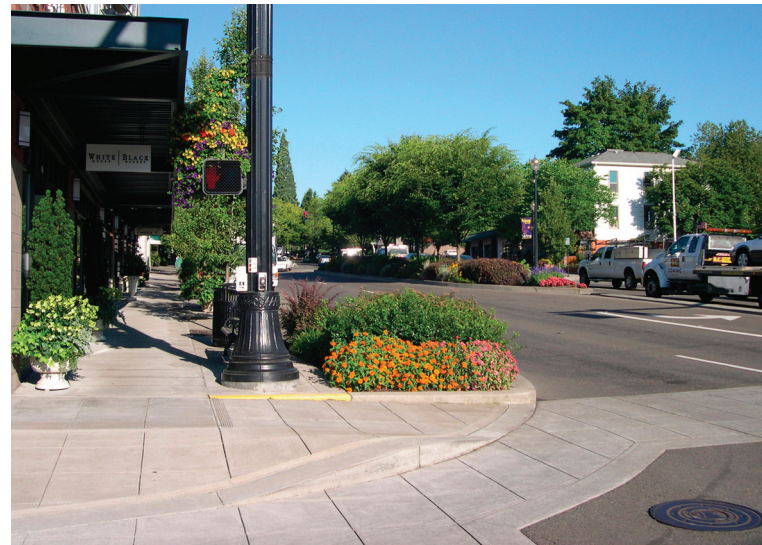
above: ADA curb ramp at street crossing
